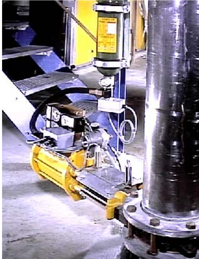
Figure 18. Explosion protection slide valve installations in a pipe
