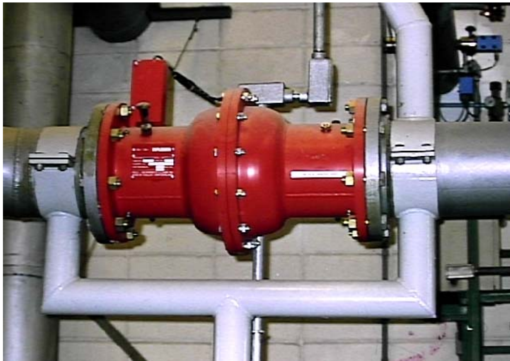
Figure 22. Self-actuated explosion protection float valve type VENTEX installed in a ventilation pipe
