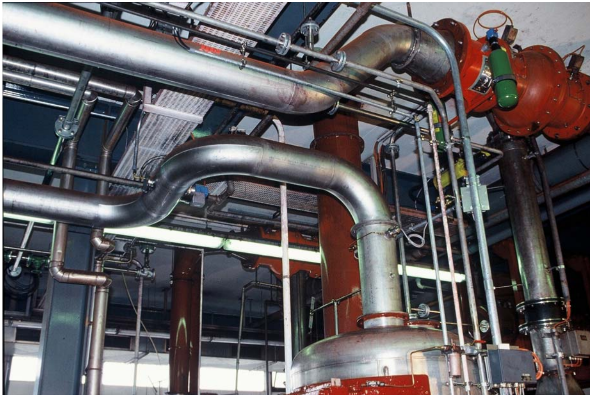
Figure 25. Externally actuated explosion protection float valve type VENTEX installed in a ventilation pipe
